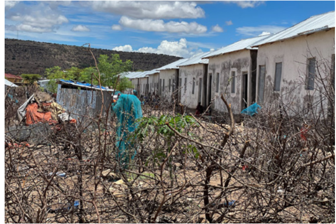
Houses constructed for relocated IDPs, Goljano woreda. Photo by Abdirahman Ahmed Muhumed
