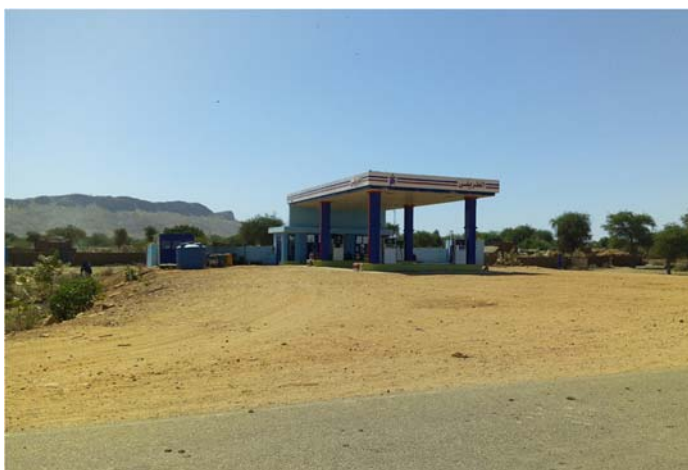
Photo: Construction of new fuel stations along the road e.g. Mornei
