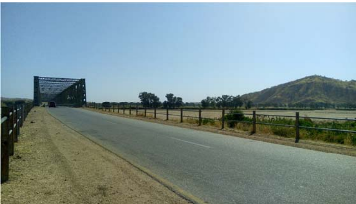
Photo: El Ingaz road: Wadi Azoom – road and bridge construction
